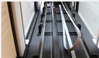
CUSTOM PAINTED MECHANICAL
